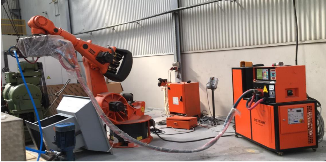
Figure 5. Induction hardening device with robotic arm
