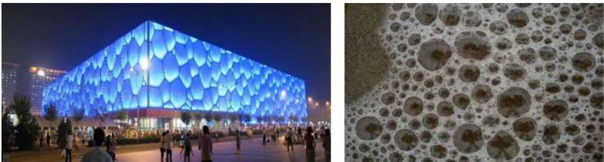
Figure 2.3. The Water Cube, Chaoyang, China, 2008, Building Views (Mirkazemi and Mousavi, 2020)
