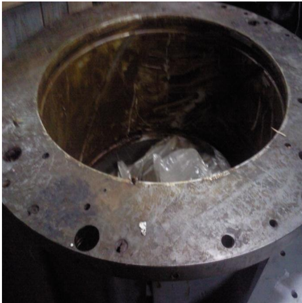
Figure 1. Turbine guide bearing.
