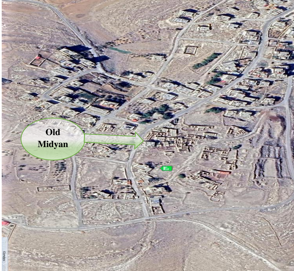
Figure 4: Aerial Photo showing the old and new Midyan
